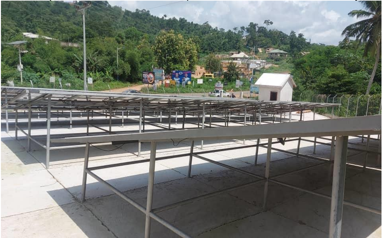
Frameworks for solar works in progress by PUMPTECH Ltd
