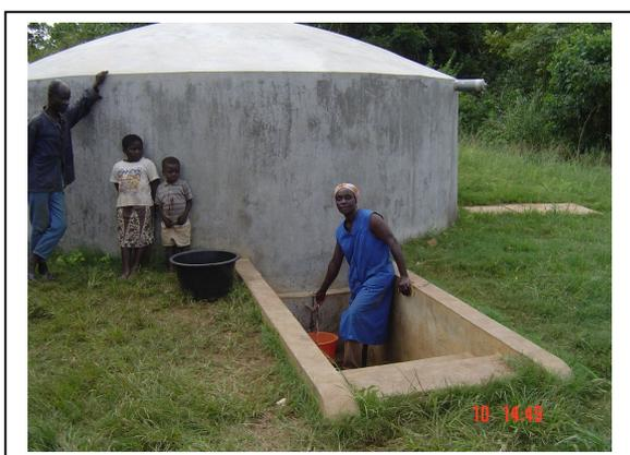
Figure 3. Rainwater facility at Ntronang showing the concrete tank, roof and eave gutter.
